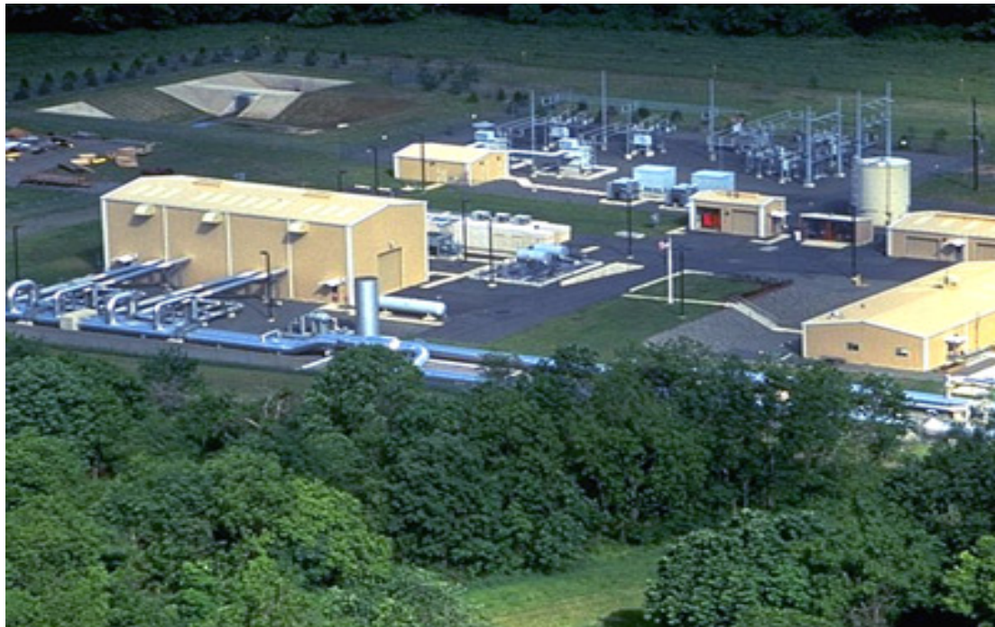
Figure 8b: Gas transmission compressor station (Source: U.S DOT PHMSA, Introduction to Pipelines )
