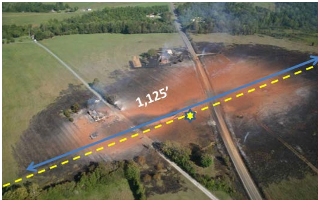
Figure 15: Appomattox, VA 2008 (Source: Pipeline Safety Trust)
