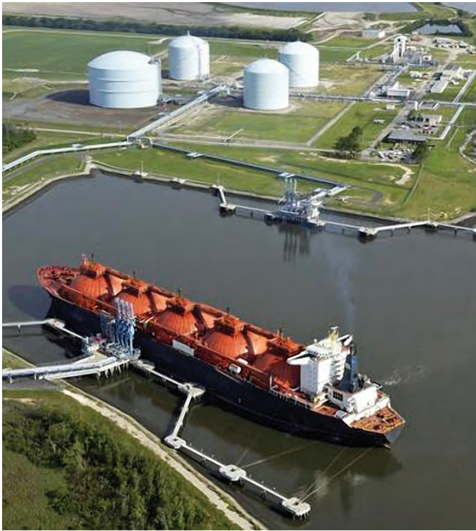
Insulated Low Pressure Storage Tanks for LNG
